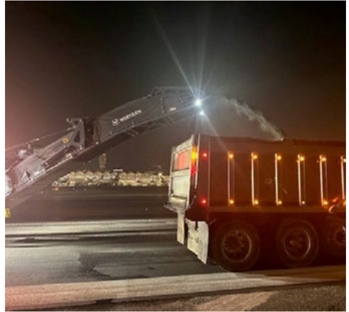
Construction vehicles worked overnight to mill and pave DCA's main runway
