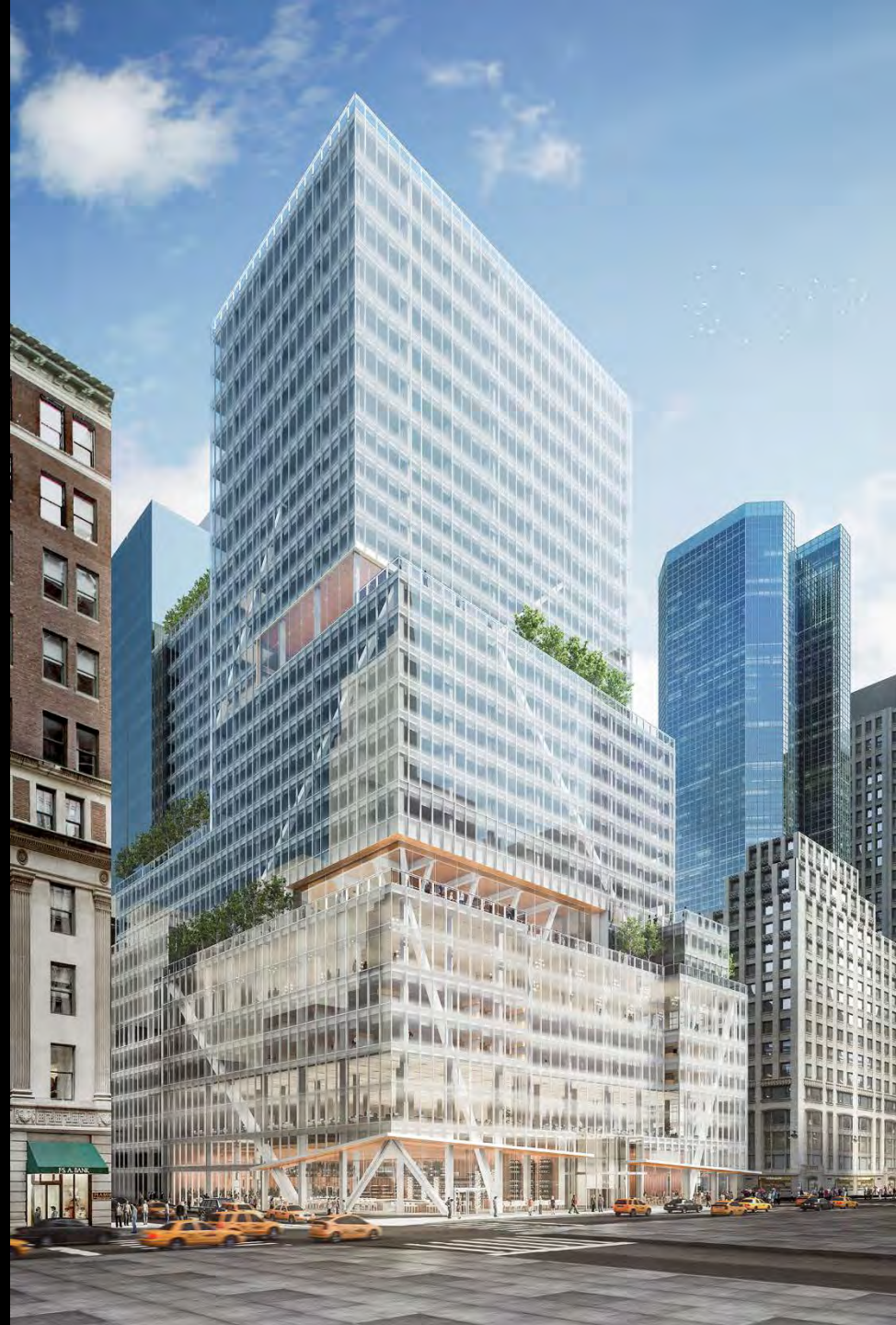
390 Madison Avenue (Under Construction) New York | L&L Holdings | 83,400 SM
